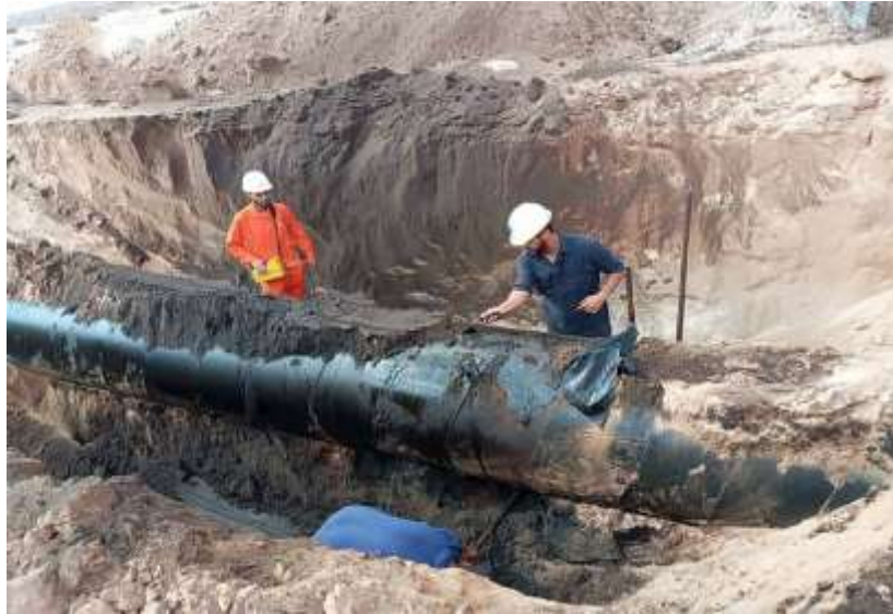
Figure 1. Corroded in the Oil Field and Coating Application Studies of 5LX42 Petroleum Pipeline
