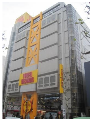
Figure 7. Cross elements applied in the building to prevent the formation of soft floors
