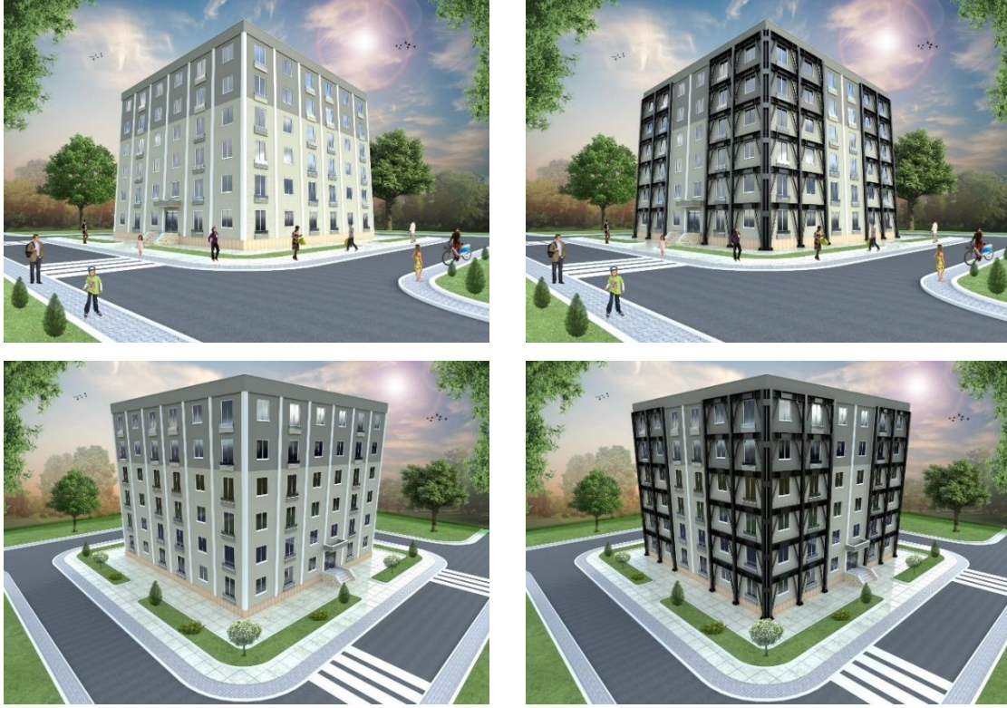
Figure 15. Building reinforced with single layer steel system
