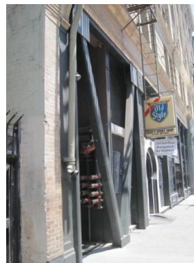
Figure 7. Cross elements applied in the building to prevent the formation of soft floors
