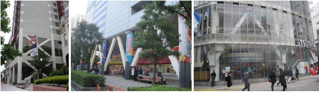
Figure 6. Cross structural elements formed on the ground floor of the building
