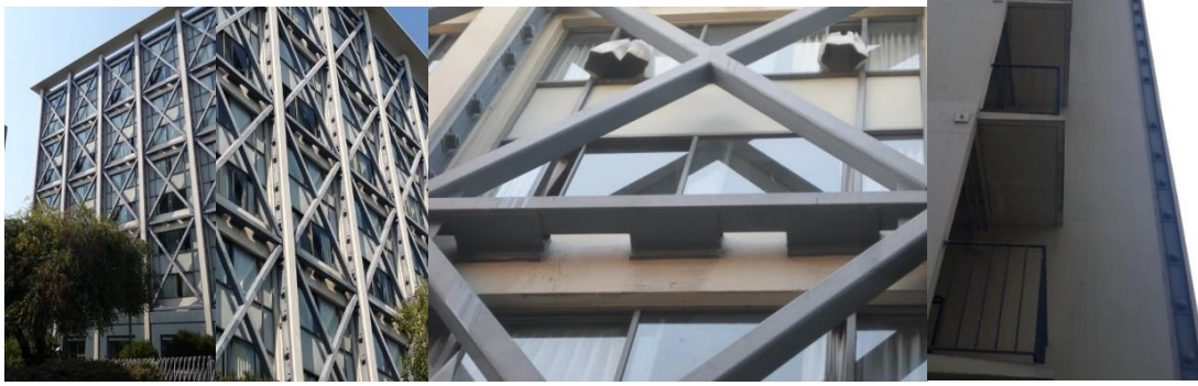
Figure 10. Example of retrofitting in a dormitory building in Berkeley
